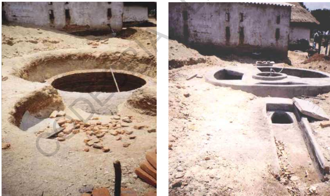
Figure 4.5: Biogas construction plant in Zimbabwe (Mavunganide Kennedy, 2005)
