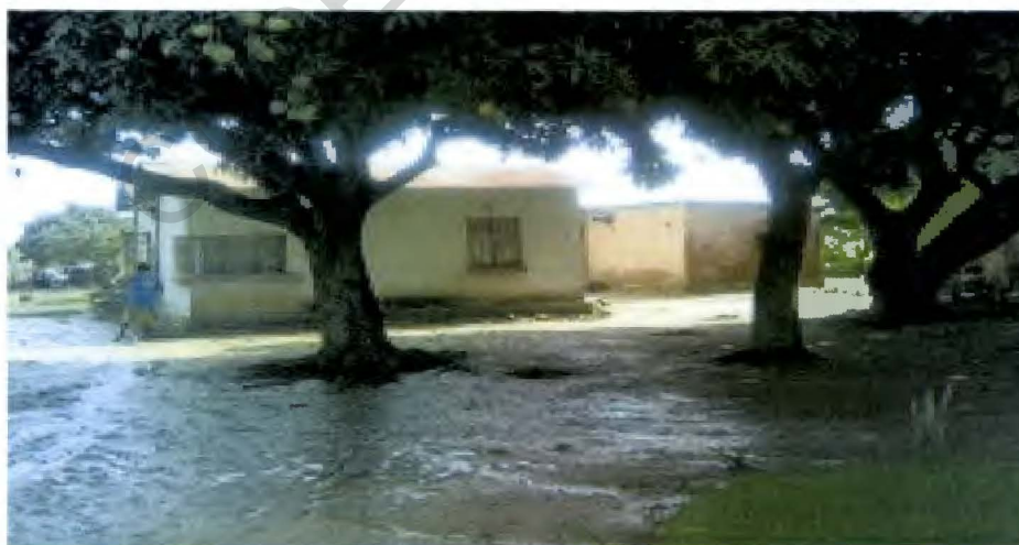
Photo 3: Water logging at Mollie's homestead after excessive rains
