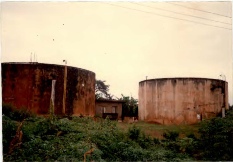
PLATE: 1: The Odenigwe Hill Reservoirs - established by and to serve the University of Nigeria, Nsukka. The combined storage capacity is 1,376,000 litres.
