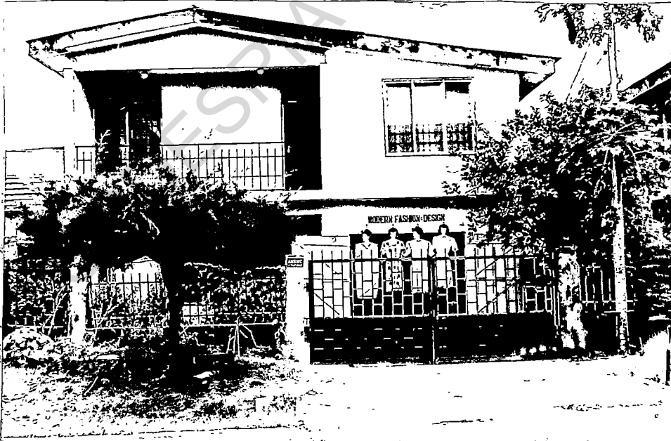
PLATE 4: Conversion of part of a Dwelling Unit to Commercial Uses. A desire for economic opportunities in housing.
