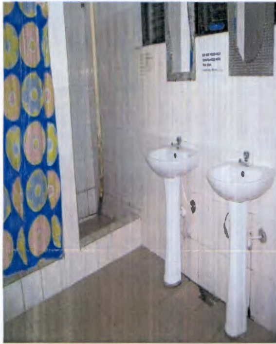
13. Facilities at the washroom of Legon Hall; too high to be used by a wheel chair user. Adaptable facilities could be provided separately for use by students with disabilities
