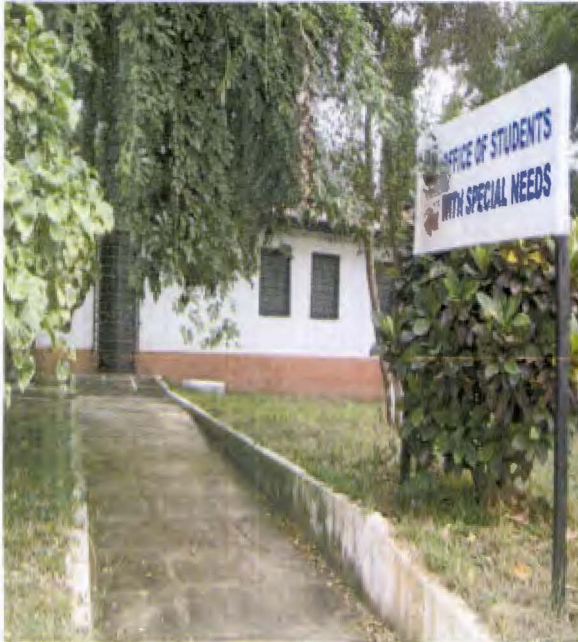
5. An accessible route to the office of students with disabilities with a rather narrow door. The narrow door could prevent wheel chair users from accessing the services of resource persons at the office
