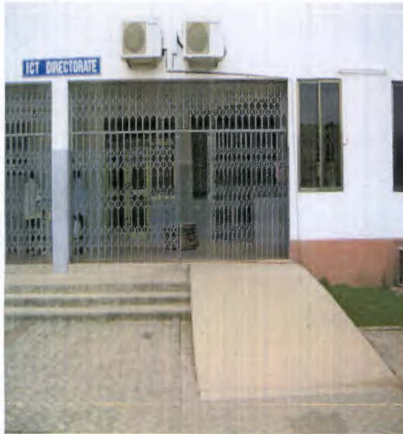
9. An accessible ramp at the main entrance of the ICT Directorate
