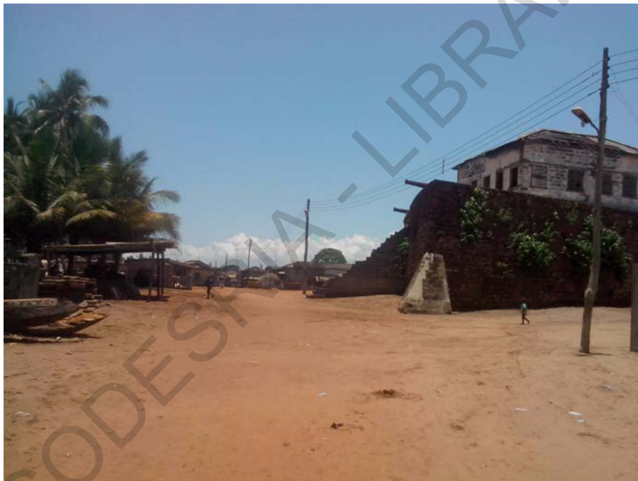
Figure 4.13: Defunct Fort (with plants on the wall) and other local structures at (British) Komenda
