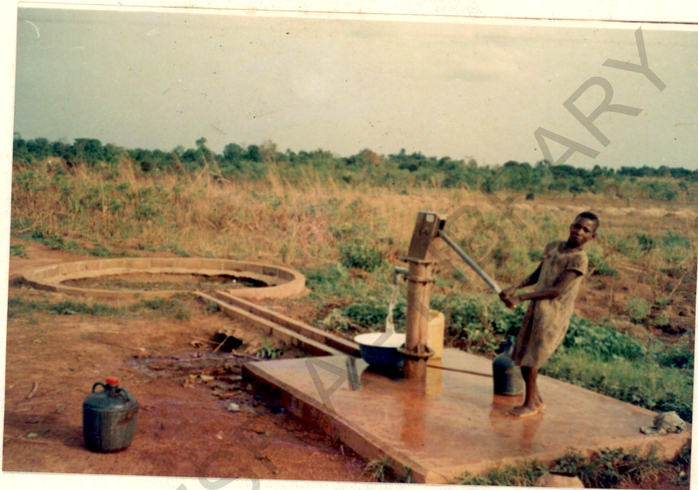
PLATE 4: Borehole with handpump by WATSAN.
