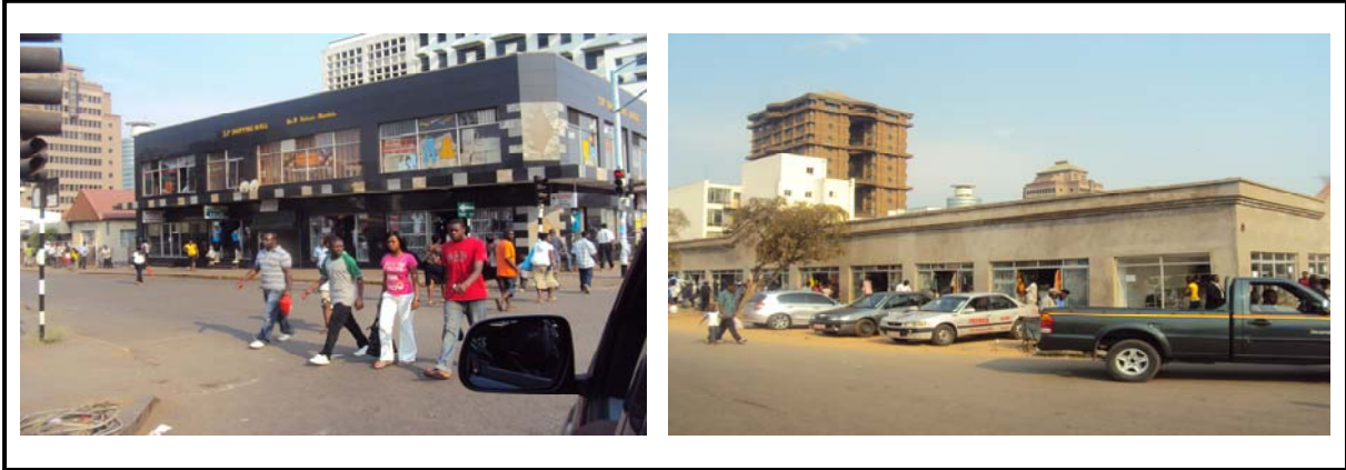
Partitioned buildings to accommodate IEEs within the CBDs during the 2000s (Harare)
