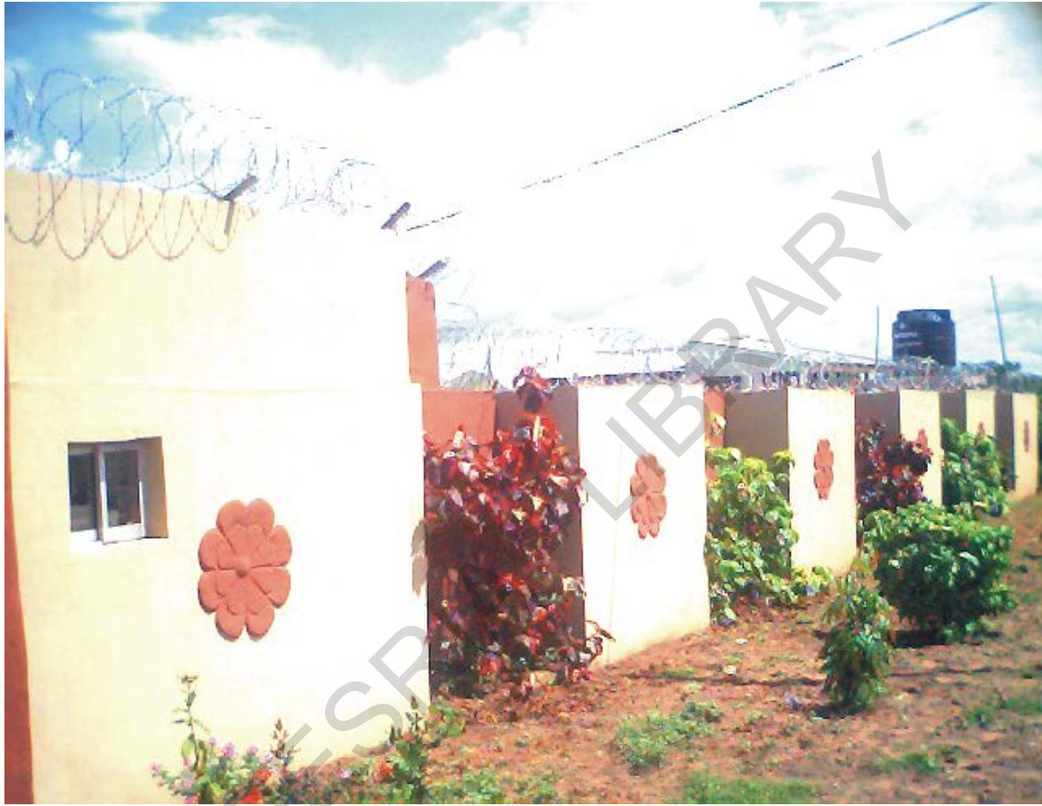
Plate 5.3: A Tall Fence with electrocuted barb wire at the tip.
