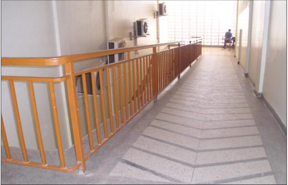
Plate 5.2: A sloping to the lower floor to enable easy movement by students with physical disability
