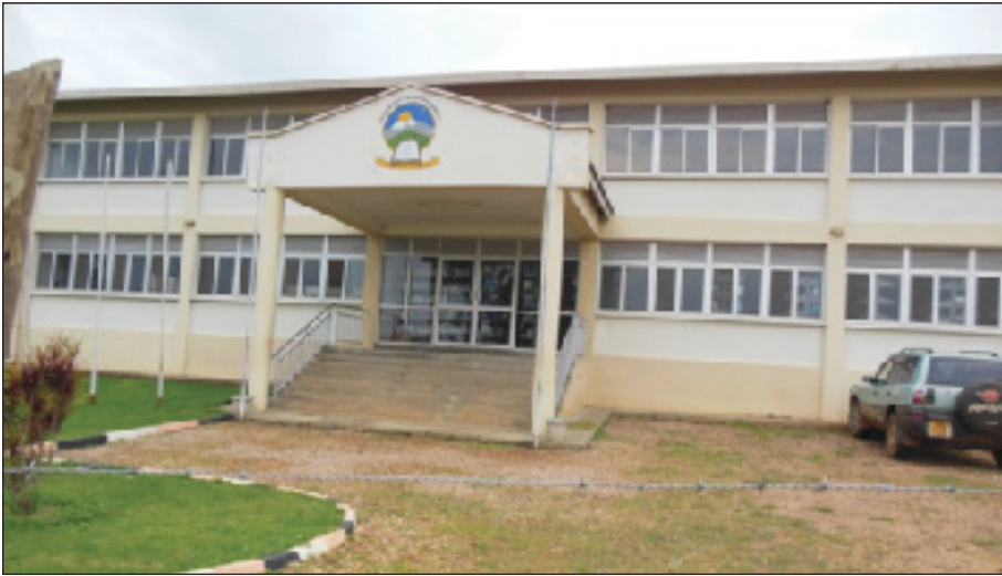
Figure 12.1: Administrative and classroom Block: Mountains of the Moon University; Fort Portal
