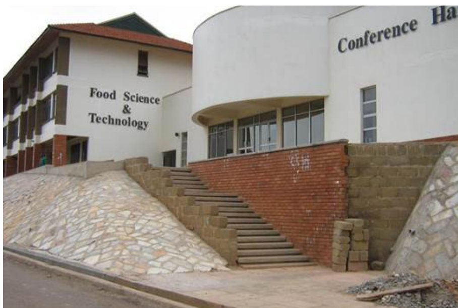
Plate 10: Food Science and Technology with Conference Centre (View from South)
