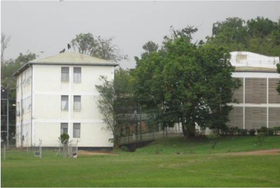
Plate 19: Faculty of Social Sciences – Community Based Rehabilitation Extension (Left), Old building (Right)
