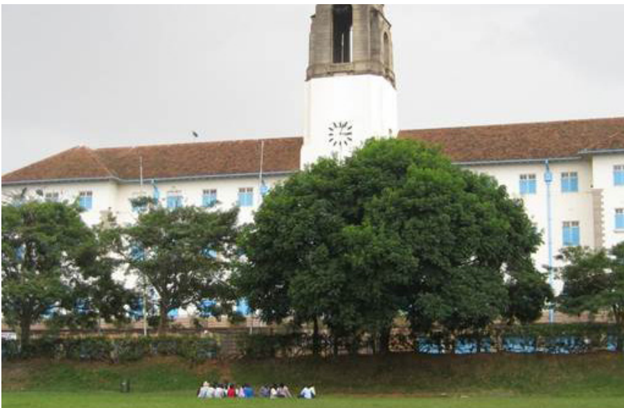
Plate 8: Main Building (Refurbished: View from the Freedom Square with Students in the Foreground)
