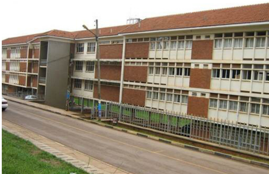
Plate 6: Lincoln House (Refurbished: Front View)
