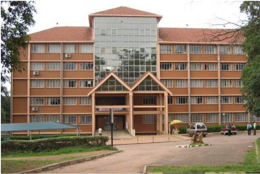
Plate 3: Senate House/Building (Front View)
