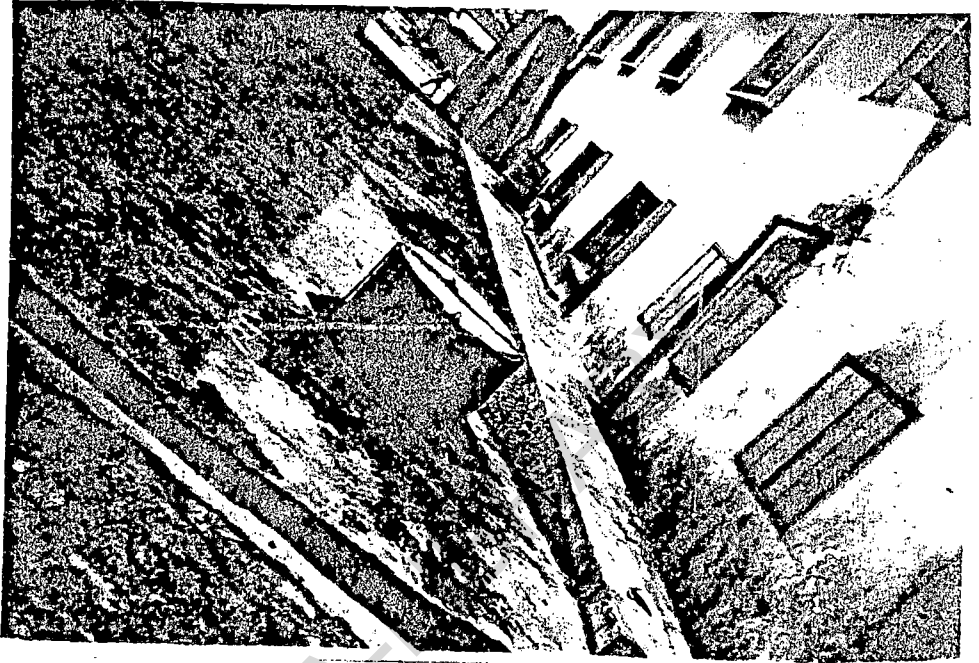
A ringed well located too close to a toilet
