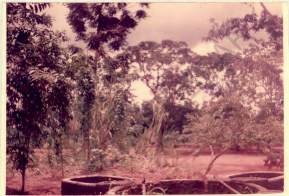
PLATE 8: An open hand-dug well (42 metres deep) in Umuosu Nsulu. Note the concrete casings and the two longitudinal iron bars where the cut bamboos with circular grooves are fitted. This well has dried up.
