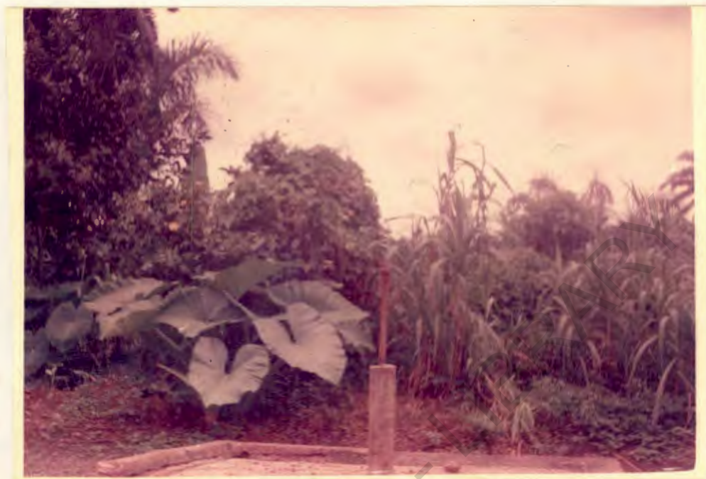
PLATE 1A: A disused standpipe in Mba village of Okporo-Ahaba Community.
