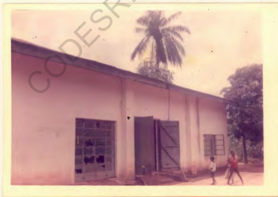
PLATE 6B: Nbawsi rural water works pump house at Umunkpeyi-Nbawsi in Nsulu community.
