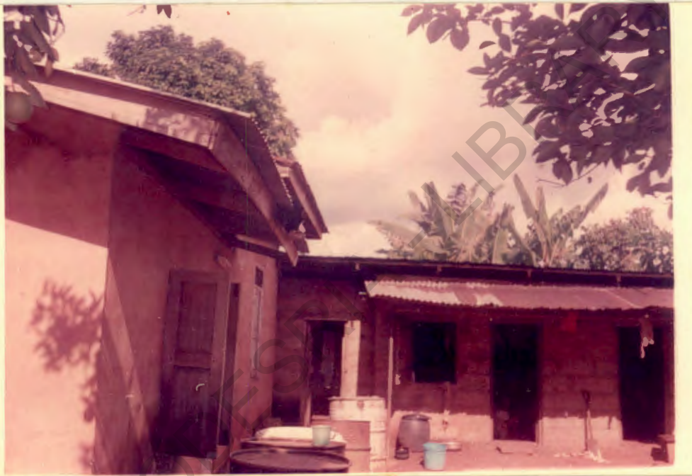
PLATE 10A: Some of the containers used for direct collection of rainwater from roofs.
