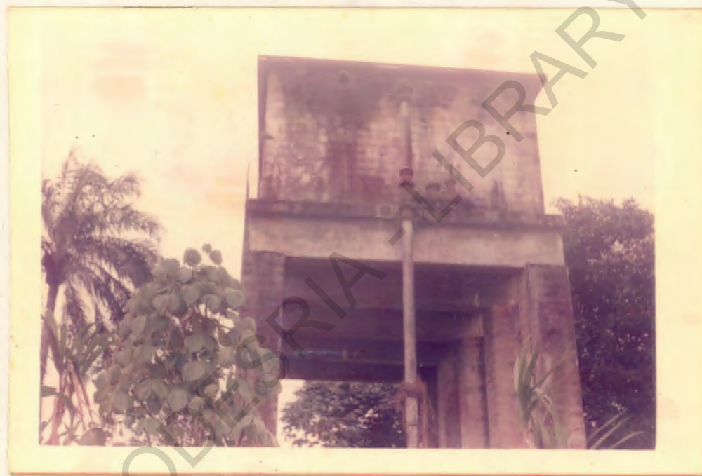
PLATE 7: Nbawsi rural water works high level service reservoir (147,000 litres) at Agburuke Nsulu.
