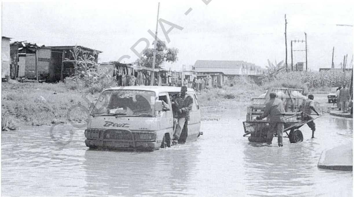
Figure 4.2: A section of a desperately in need of maintenance road in Nairobi's Eastlands in the 1990s (photo Courtesy of Antony Kaminju).
