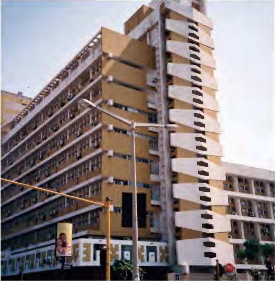
▲ Figure 9.3 Ministry of Health building, Maputo
