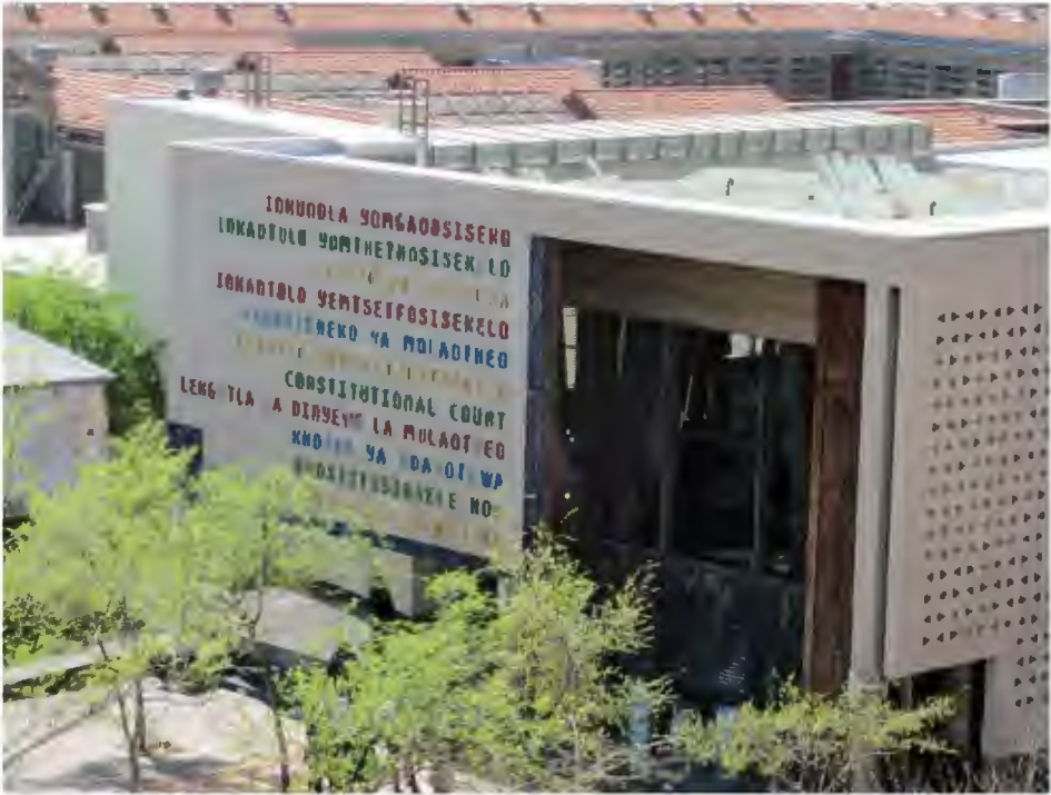
Figure 10.5 Constitutional Court building, Johannesburg
