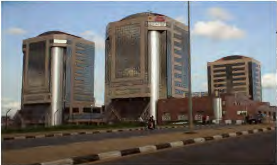
Figure 6.3 Nigerian National Petroleum Corporation Towers, Abuja
