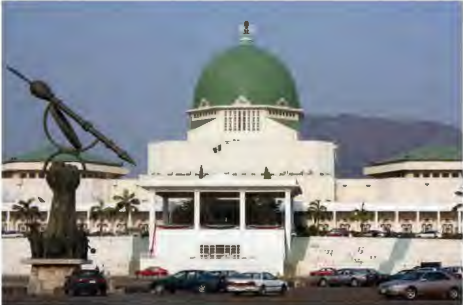
Figure 6.1 National Assembly, Abuja
