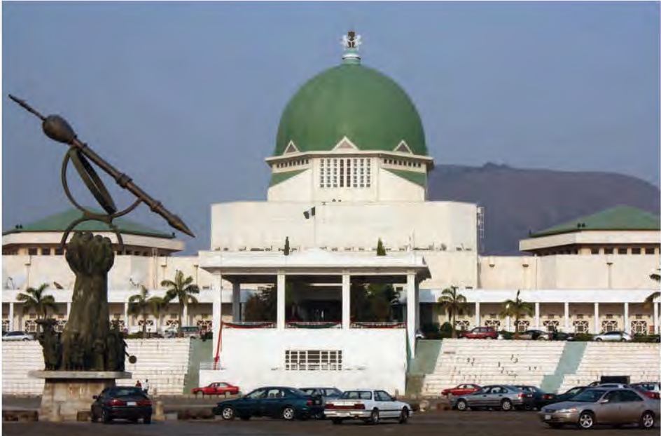
Figure 6.1 National Assembly, Abuja
