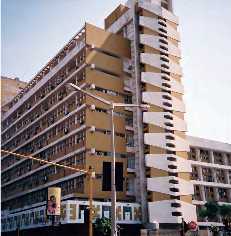
▲ Figure 9.3 Ministry of Health building, Maputo
