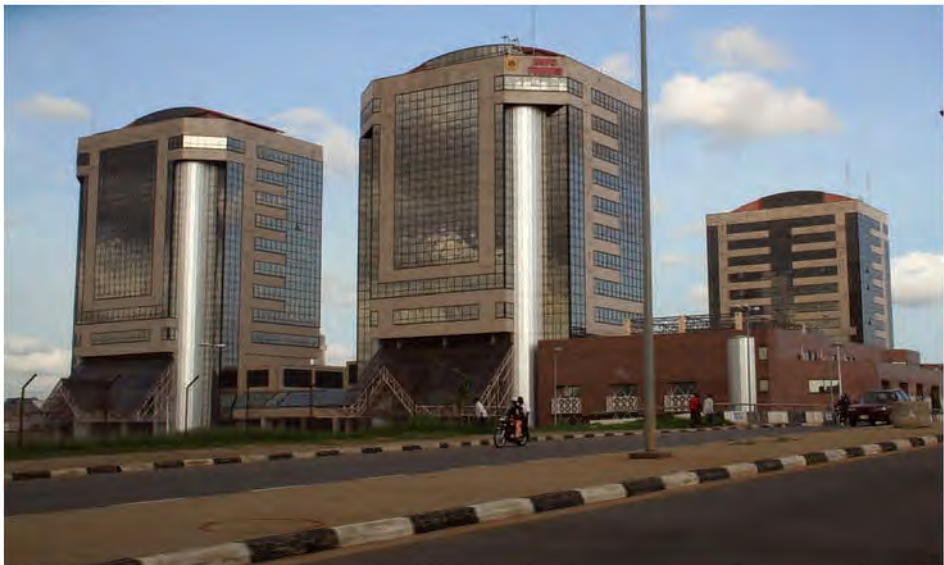
Figure 6.3 Nigerian National Petroleum Corporation Towers, Abuja
