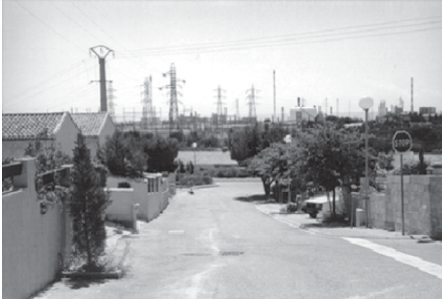
7. Hamlet of Lavéra (Martigues, July 1996). Photograph: Franck Pourcel
